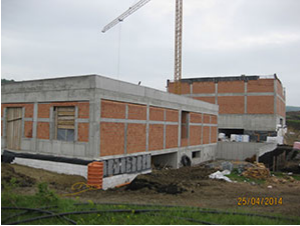
CREIC works progress in April 2014.
